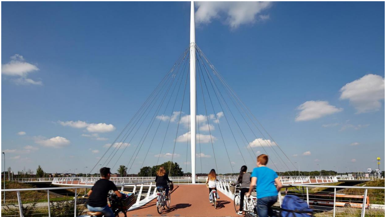
Hovenring Cyclist and Pedestrian Bridge, Eindhoven, the Netherlands 1
